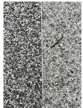
Movement joint with applied resin bound surface.
